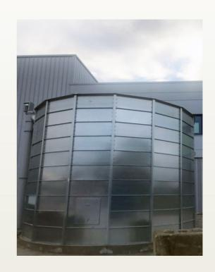
We installed a 90m3 wood chip silo made from galvanised steel and a loading auger capable of transporting wood chip from a tipper truck into the silo at a speed of 45m3 per hour.
