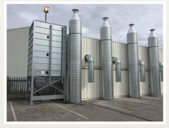
Each silo was to be placed beside two 40 foot shipping containers stacked on top of each other and fed a total of 4 x 50 kw chp boilers which provided heat and power to businesses in the industrial estate as well as doubling as a testing centre allowing Entrade engineers to experiment with using different waste streams as fuel.
