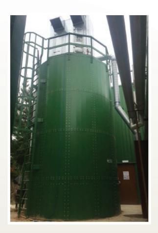
As this filter unit had to be serviced and maintained regularly a roof access ladder and safety railings were also provided. The silo itself was a 60m3 cylindrical store measuring 3.5m in diameter X 6m high. As the site had no access for lifting equipment the silo had to be brought to site flat packed and built in situ. As per customer request it was also powder coated leaf green in order to match the colour of the building it was sited next to.
