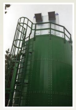
Significant engineering challenges also existed on the extraction end of the silo where we were asked to provide a **horizontal agitator type screw auger system 1.2m from ground level** to feed into a secondary boiler feed screw which was already installed on site. A **precise feed rate of 308kg per hour** had to be achieved in order to integrate the two augers.
