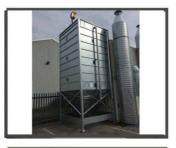
60 Degree hopper base allows mass flow of pellets and reduces the need for cleaning silos
