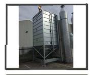
60 Degree hopper base allows mass flow of pellets and reduces the need for cleaning silos
